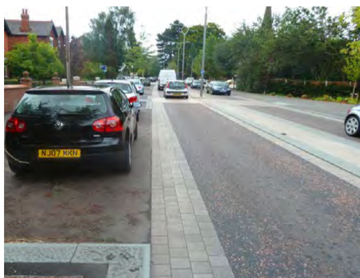
Central Median - Introduce a near flush central median to reduce carriageway space (tarmac) and reduce traffic speed, whilst allowing informal pedestrian movement and protected parking
