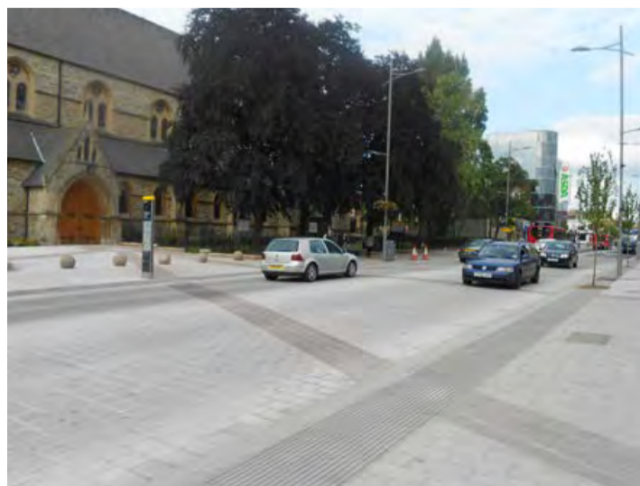
Flat top table - Flush flat top speed tables linking lateral public spaces at key nodes and gateways
