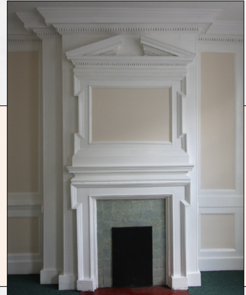
8f: A fine 'eared' fire surround and overmantle with a broken pediment. This is the centrepiece of a panelled room in a townhouse of c.1740. It is the best example of its type in the Maldon District. Great care must be taken not to disturb this joinery through work such as re-wiring.
