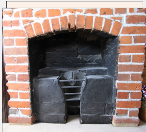
8g: An original bedroom fireplace incorporating hobgrate in a Georgian cottage of c.1760.
