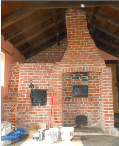
8h: The interior of a Brewhouse attached to a listed farmhouse. In the back of the fireplace can be seen the doors to a bread oven. To the left-hand side is a warming copper. Such features provide a valuable record of the routine activities which structured life in vernacular houses.
