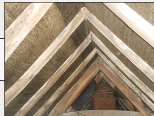
12c: When each pair of rafters is separately jointed and pegged at the ridge, this is normally an indication the roof pre-dates c1800.
