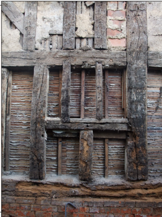
FIG. 5: 16th-century timber-framed structure exposed during re-rendering at Bridge Farmhouse, Tollesbury.
