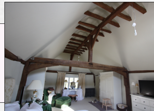
12a: This is a late example of a crown-post roof. The crown post is the vertical timber standing on top of the tie beam. The top of the crown post and its two braces are connected to a central 'collar purlin'. Most houses dating from c.1300-c1550 had this type of roof.
