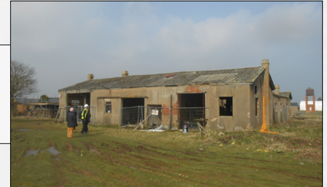
FIG. 4b: The Officers' Mess at Stow Maries Great War Aerodrome photographed in 2016, now listed grade II*. Consent has been granted to restore this elevation in accordance with the old photograph.
