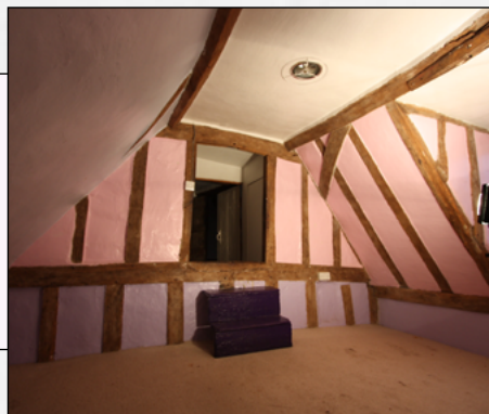
12b: Crown-post roofs fell out of use during the second half to the 16th century, and were superseded by side-purlin roofs. This is an example of a 'clasped' side-purlin roof in a house dating from the late-16th century. Note the arched wind braces which were common before the 18th century.
