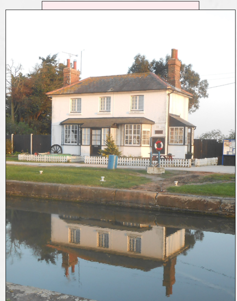
FIG. 7: Lock House in Heybridge Basin.
