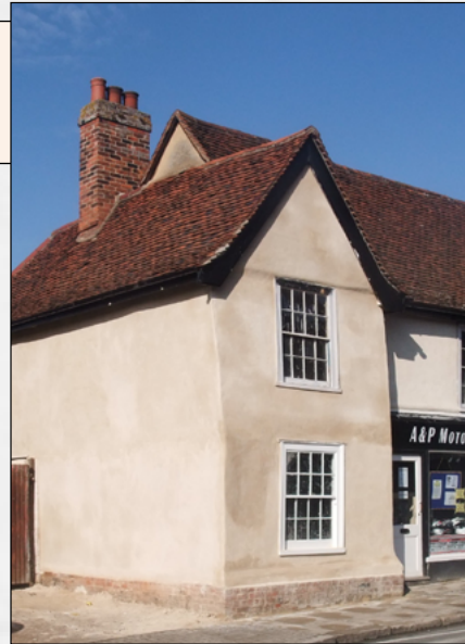
FIG. 8 (a - n): Examples of special features in listed buildings in the Maldon District
