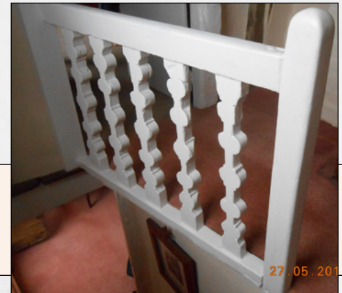
8i: Stair bannisters in a grade II listed cottage dating from the late-17th or early-18th century. The splat balusters are of an unusual ovolo-moulded design, and may be recycled. The rustic character of this feature reflects the humble status of the cottage.
