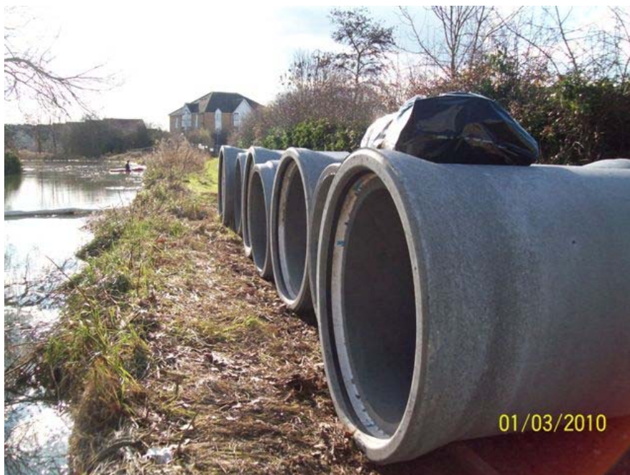
Figure 5.5: Canal Chunker repairs
