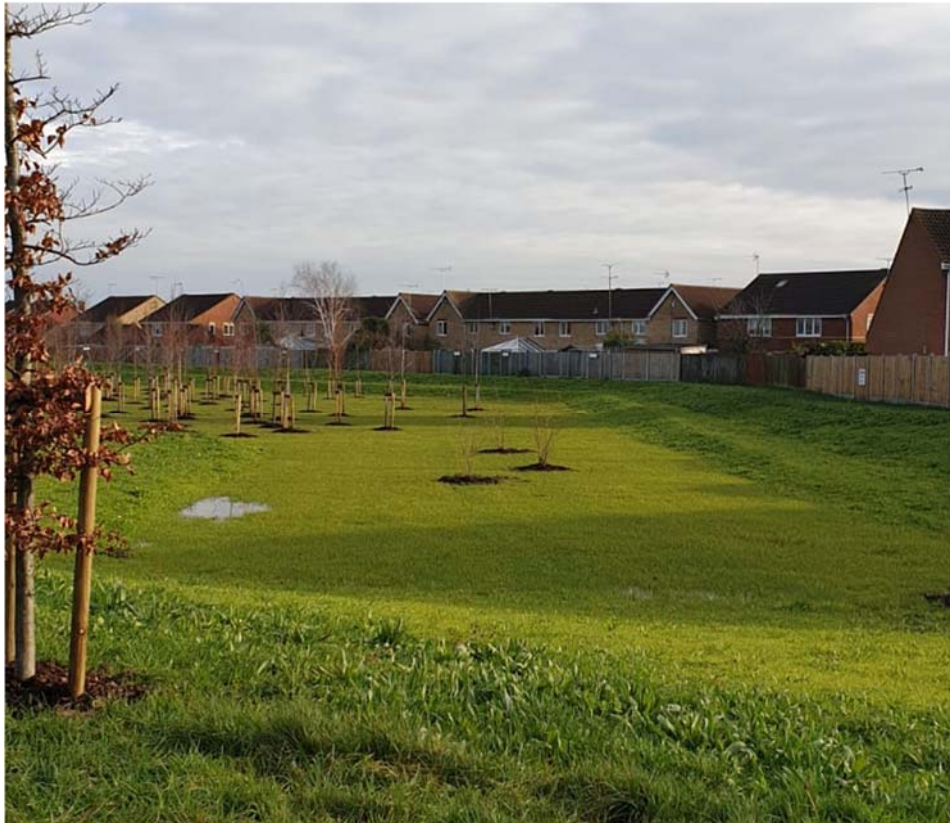
Figure 6.9: A grassed; below-ground detention basin created as part of the ECC Brickhouse Farm flood alleviation scheme in Maldon
