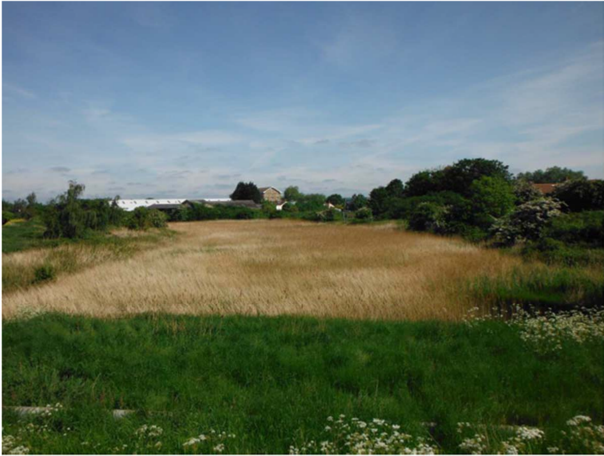
Figure 6.8: View from Upstream of the Sadd's Dam Embankment that is within the Causeway Regeneration Area
