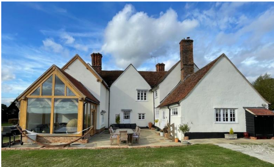
The rear (east) elevation of Hazeleigh Hall with new extensions to the left
