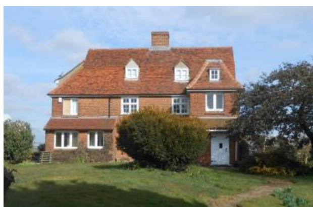
High House in 2015, prior to restoration
