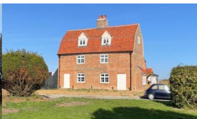
High House in October 2022, after restoration. Later front and side extensions have been removed to re-establish the building's original form.
