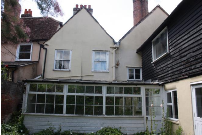
Above: The rear elevation prior to renovation.
