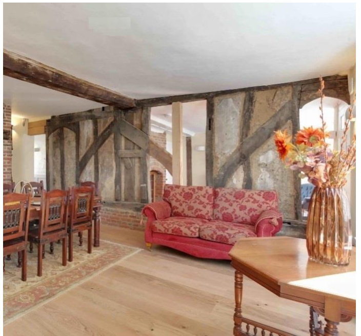
A medieval wall in the hall with two original arched doorways (the left one blocked). The ceiling was introduced into the hall as part of a major refurbishment dated by tree-ring analysis to c. 1578.
