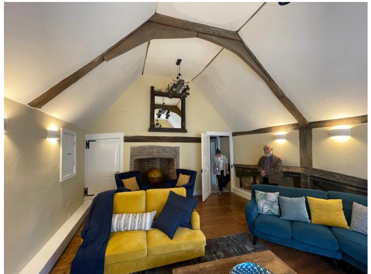
The hall chamber in 2023. A later ceiling was removed to re-expose the roof truss of c.1578.
