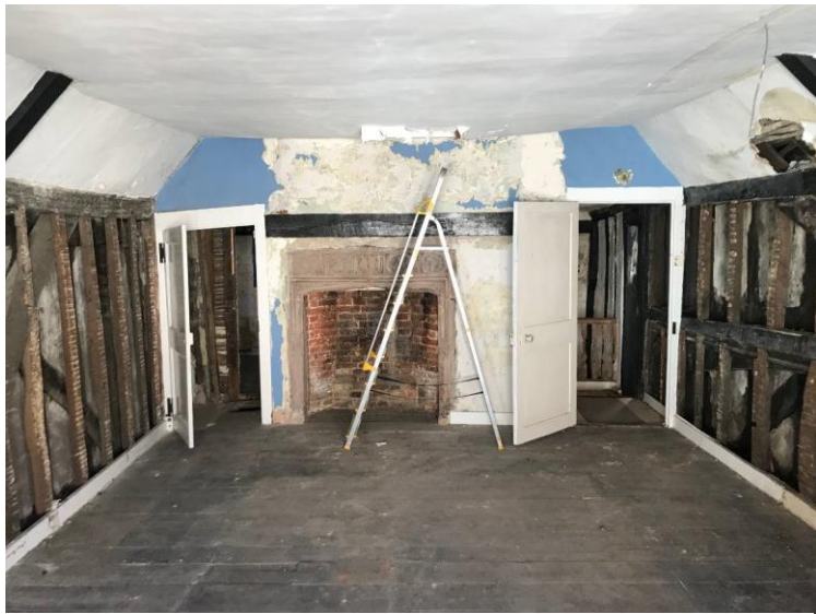
The hall chamber during refurbishment.
