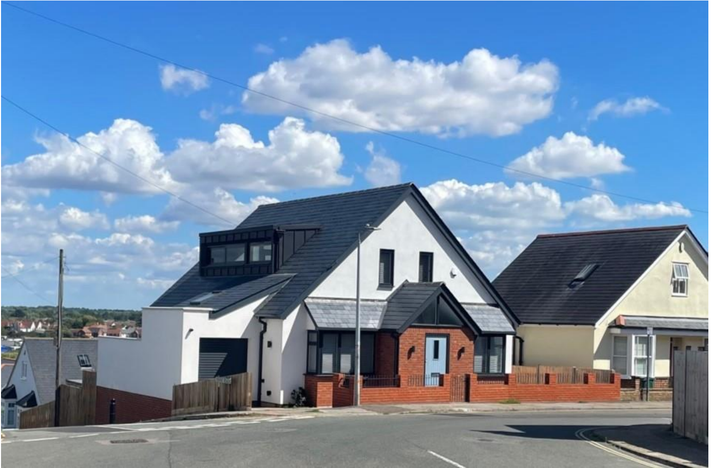
The front elevation of 66 Victoria Road, Maldon
