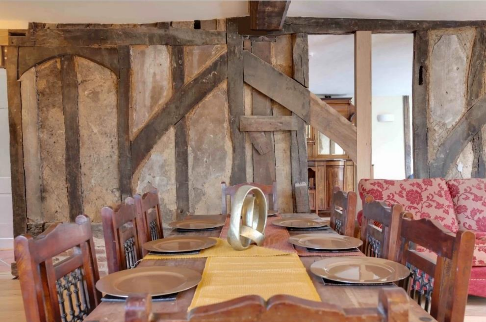
An early 15 th -century wall inside 4 Silver Street, Maldon, recently uncovered and conserved. Interventions were kept to a minimum to preserve the unique wall's patina of age. Photograph by Angela Westgarth.
