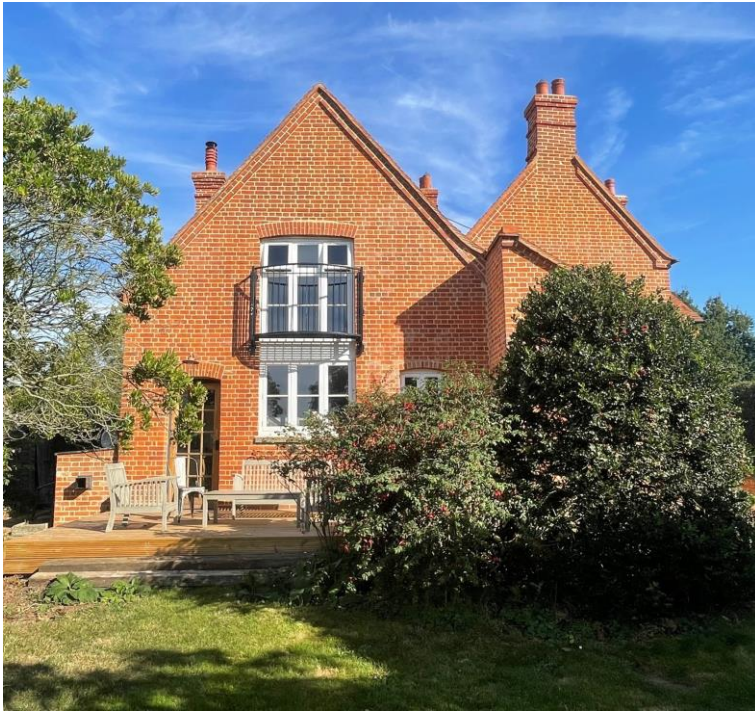
The rear elevation of Old School House
