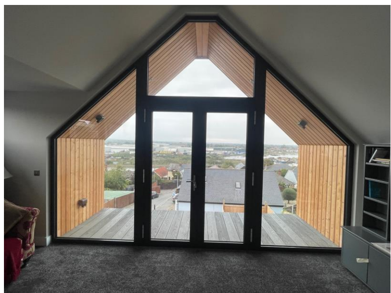
The rear first-floor window and balcony
