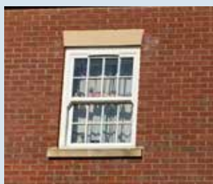
Sash window and lintel details
