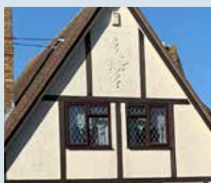
Mixture of render and timber
