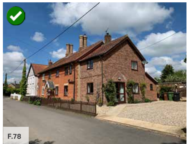
Figure 78: Positive example of side extension which complements the scale of the existing property, somewhere in the UK.
