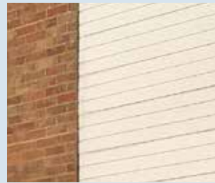
Mix of red brick and timber cladding
