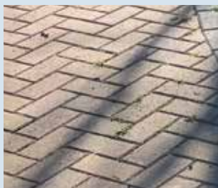
Herringbone brick paving
