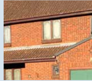
Red pantile and chimney stacks
