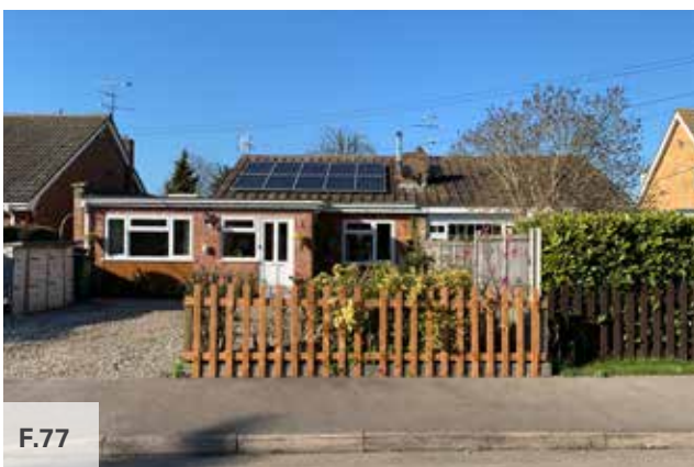
Figure 77: The original building should remain the dominate element of the property. The front extension is not of a sympathetic scale. The flat roof should be avoided in any future developments.
