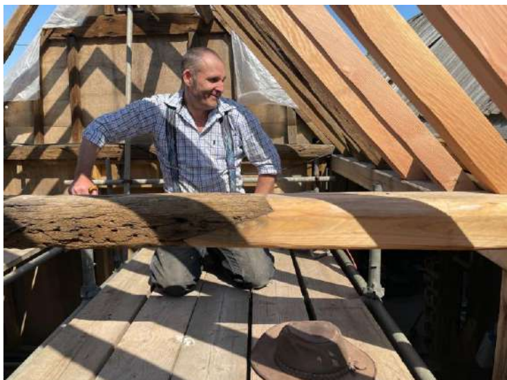
Carpenter Andrew Blowers admiring his timber-frame repairs in June 2023.
