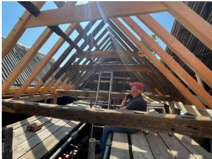
Owner David Thorpe contemplating the restored roof in June 2023
