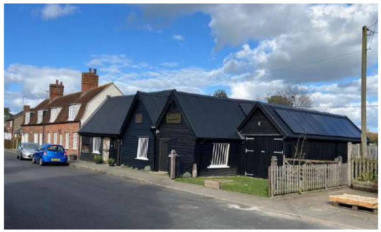
The Forge in March 2026, following renovation
