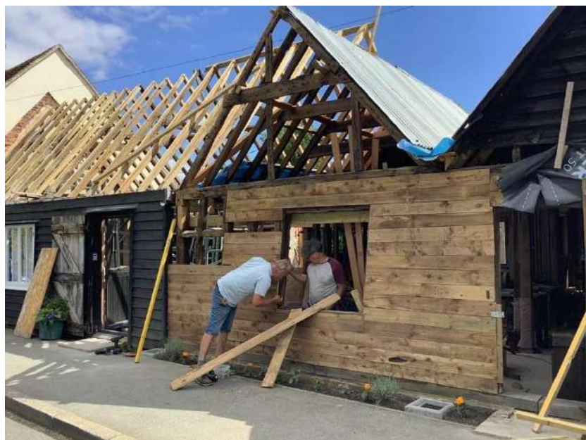
Tony Baker and Lee Robinson replacing cladding in 2024.
