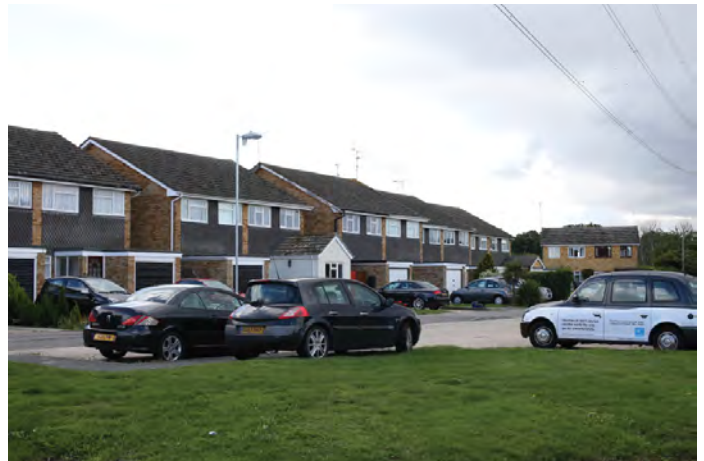
Exposed Car Parking - 1m high Hedging could better screen this from view
