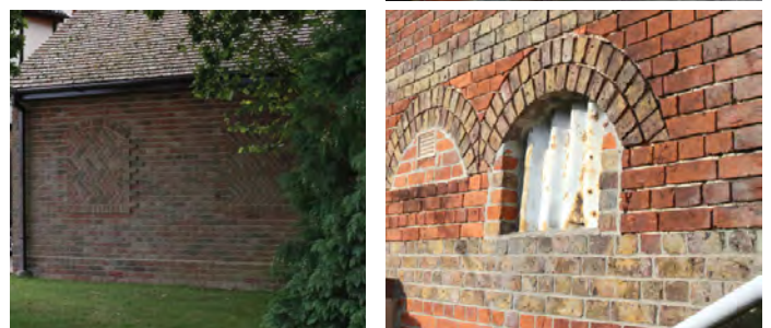
Brick and Render combined, Original 1930 Herringbone Brick Detail, Modern Herringbone Brick Detail, Window Brick Detail
