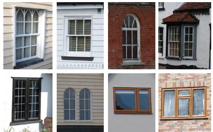
Timber Sash Window, PVC Sash Window, Timber Arch Window, Bay Window, Timber Casement Window with oblong lead detail, PVC Arch Window, Light Brown PVC Casement Windows
