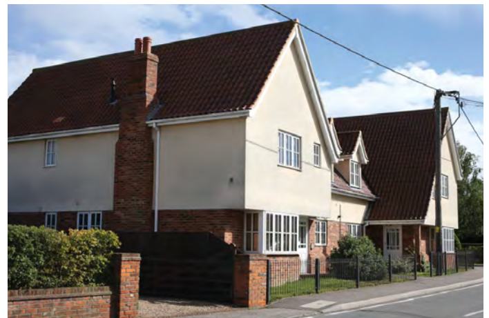
Hamilton Court Flats built in 2000s
