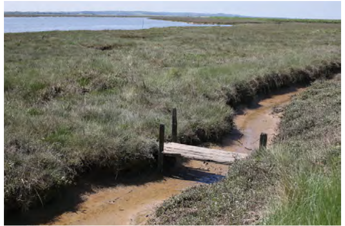
Timber bridge within mudflats of the River Crouch
