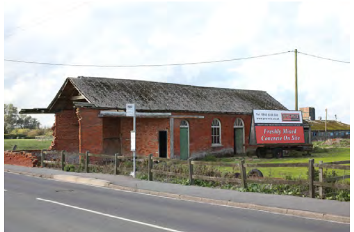
Part demolished - original outbuilding of Mansion House Farm
