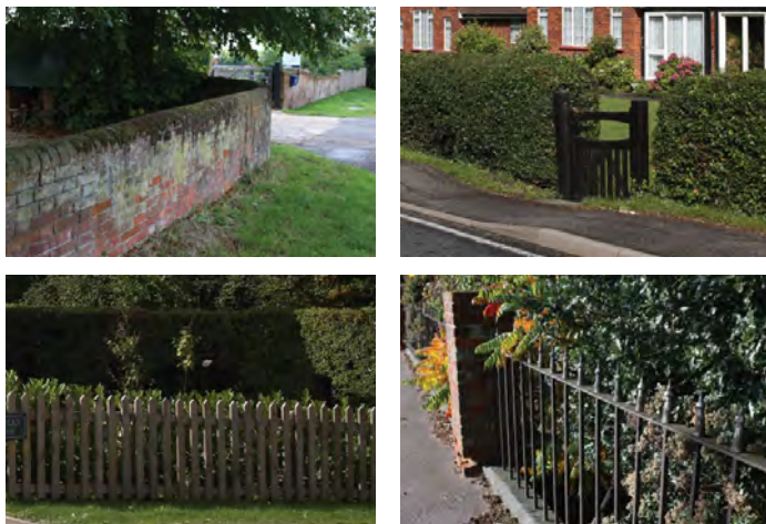
Brick Wall, Indigenous Hedge, Picket Fencing, Red Brick and Metal railings
