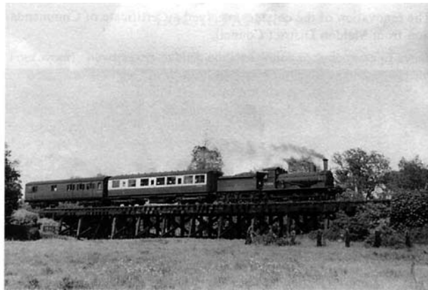
The Viaduct in use May 31st, 1958 Reproduced by permission of Colin Hogg, courtesy MIKE ESAU
