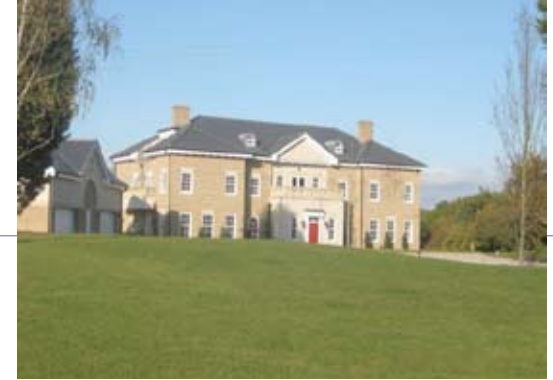
Fig 3H New Witham Road Mansion
