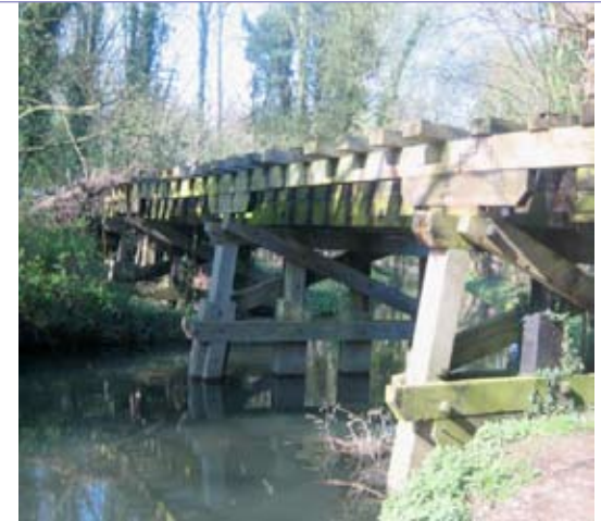
Fig 2F Timber Trestle Viaduct
