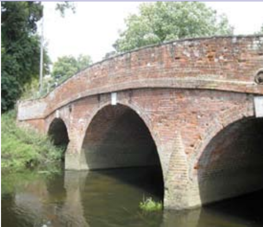
Fig 1A Blackwater Bridge
