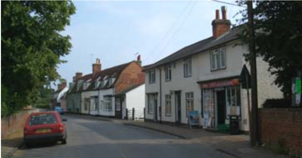
Fig.27 East side of High Street
