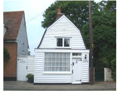
Fig. 10 Weatherboarding
