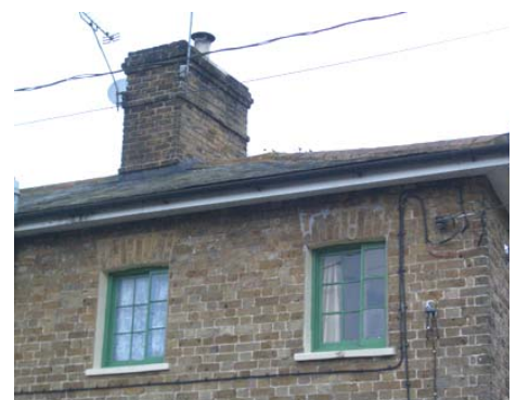
Fig. 14 Chimneys, brick details and original horizontally sliding sash
