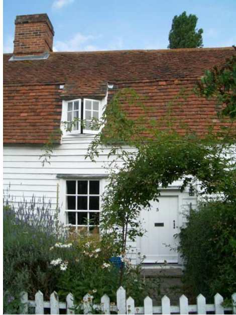
Fig. 15. Typical details: weather-board, tiled gambrel roof, a narrow dormer and picket fence.
