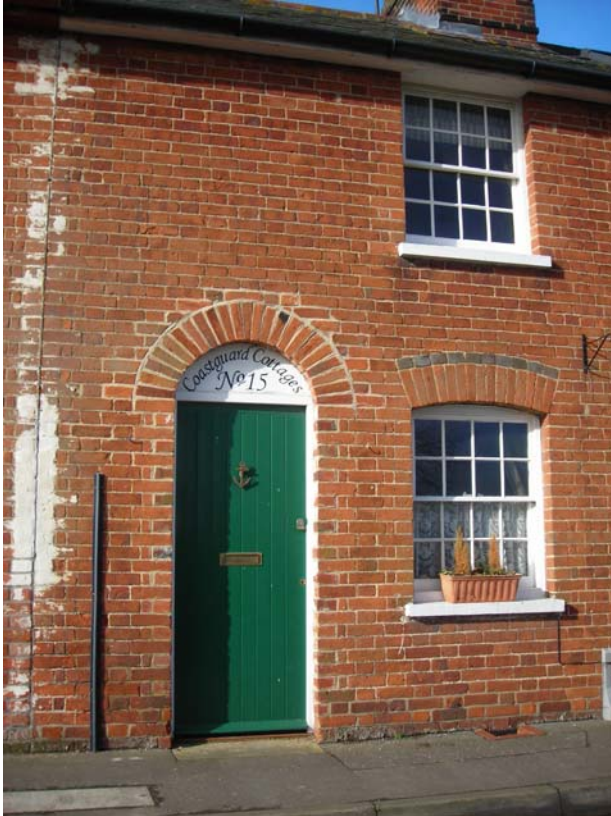
Fig. 19 Coastguard Cottages, a good traditional elevation with unpainted red brick in Flemish bond, small-paned timber sashes and a simple boarded door.
