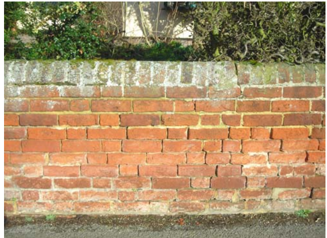
Fig. 21 Traditional brick boundary wall, no. 6 Head Street.
