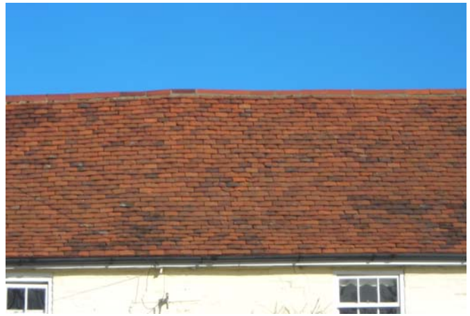
Fig. 20 Handmade plain clay tiles, no. 2 Head Street.
