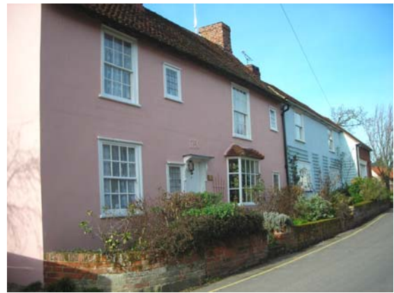
Fig. 48 Nos 2-4 Fish Street.
