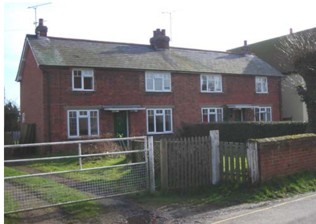
Fig. 58 Nos 9-11 Fish Street.
