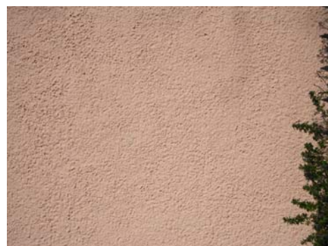
Fig. 18 Rough painted render on a timber-framed building, no. 2 Head Street.
