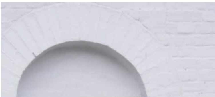
Fig. 23. Painted brickwork showing door arch
