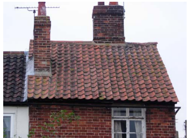
Fig. 27. Handmade red clay pantile
