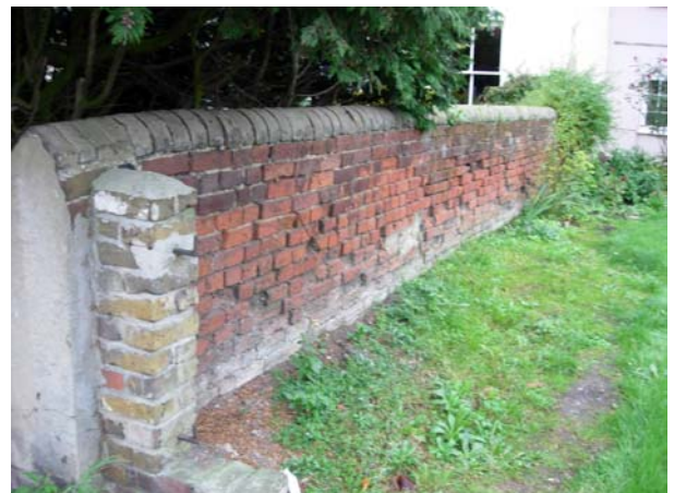
Fig. 38. Red brick wall with half-round capping bricks
