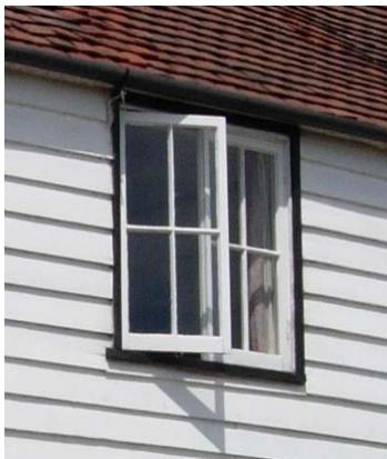
Fig. 29. Side opening timber casements
