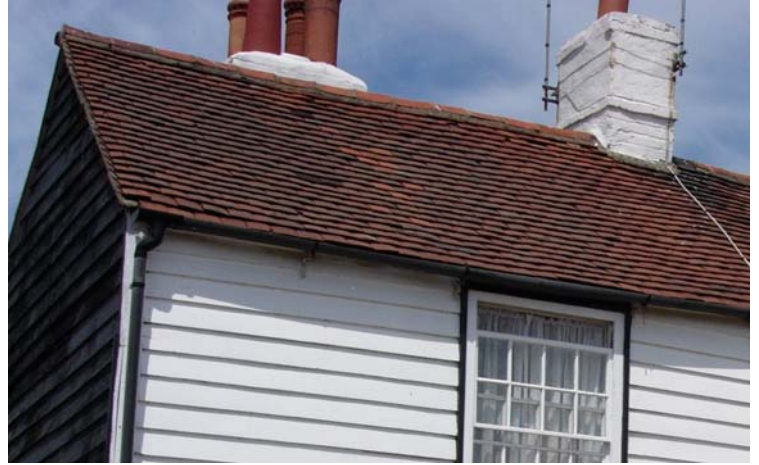
Fig. 25. Handmade plain tile roof
