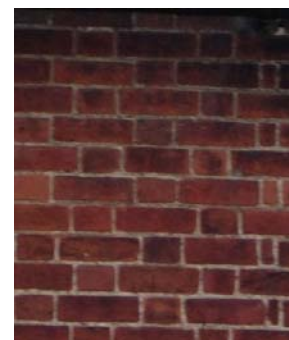
Fig. 24. Flemish bond red brick
