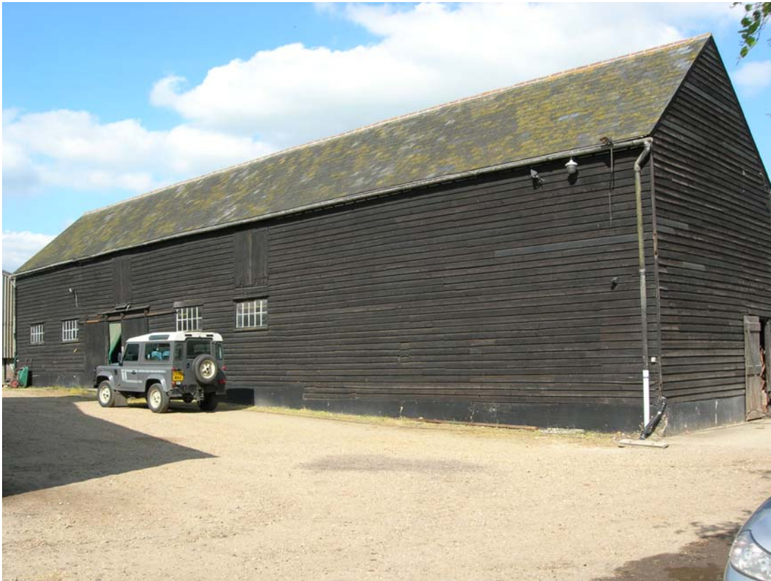
Fig. 51 Barn still in farm use
