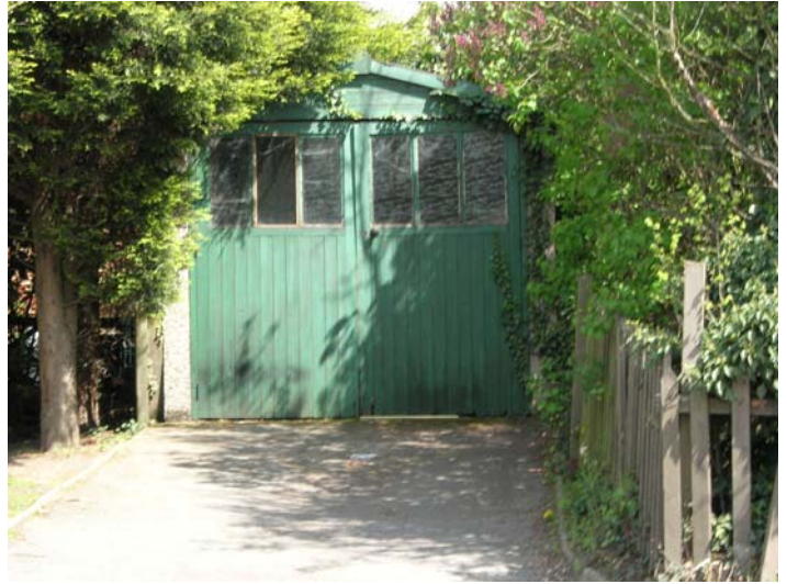
Fig. 40 Garage between Chesterton and the Old School House
