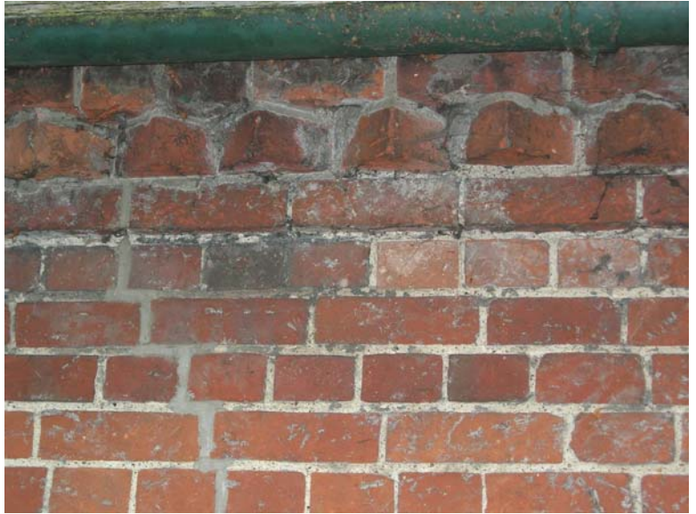
Fig. 10 English bond brick detail on village hall below a sawtooth course at the eaves.
