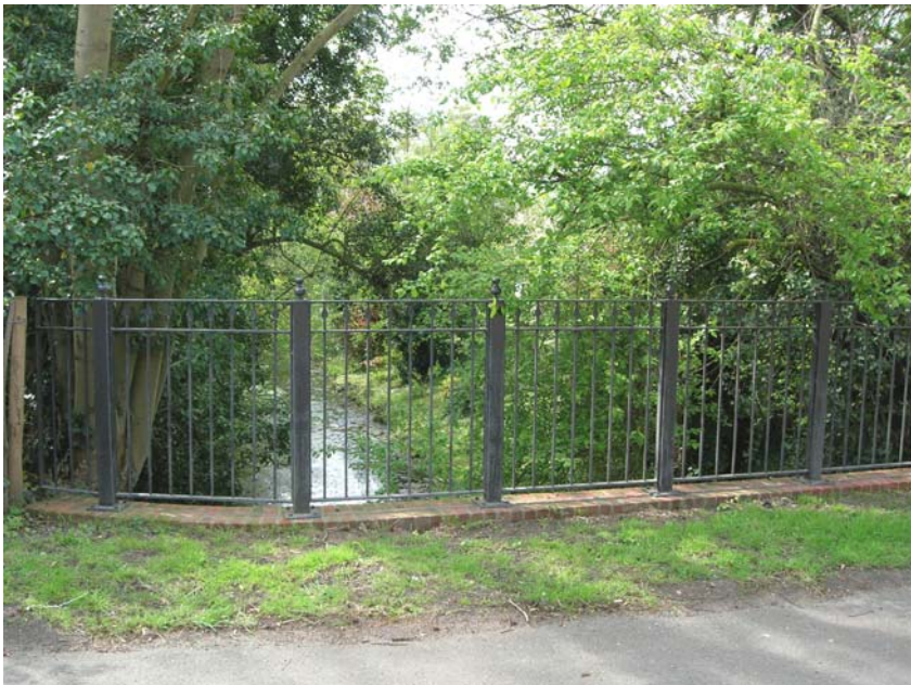
Fig. 29 Railings and wall above Langford Cut
