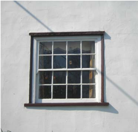
Fig. 22 Traditional timber small paned sash window, The Bell.
