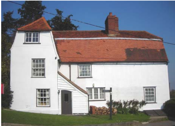
Fig. 34 The Bell, showing medieval hall house range.
