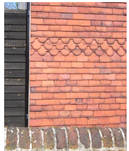
Fig. 21 Decorative tile hanging on The Old Bakery.
