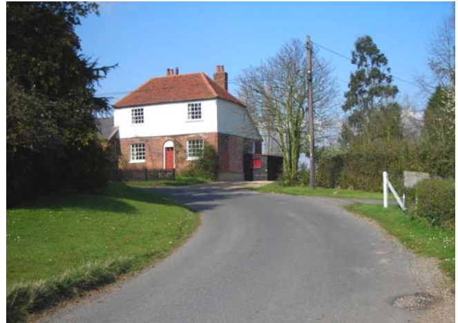
Fig. 10 Eveleigh House looking north.
