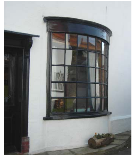
Fig. 26 Original 18th century shop window, The Old Gate House.
