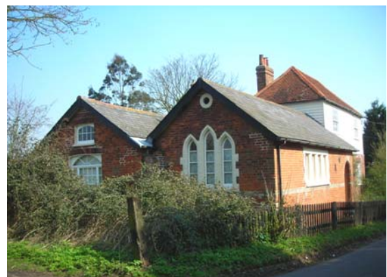
Figs. 32, 33 Eveleigh House, with the brick classrooms (bottom).
