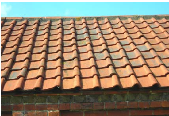
Fig. 25 Clay pantiles used on a traditional farm building at Purleigh Hall Farm.
