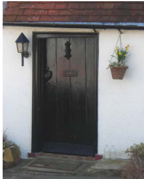
Fig. 23 Traditional timber boarded door, the Old Gate
