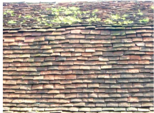
Fig. 24 Handmade double cambered clay tiles on the roof of
