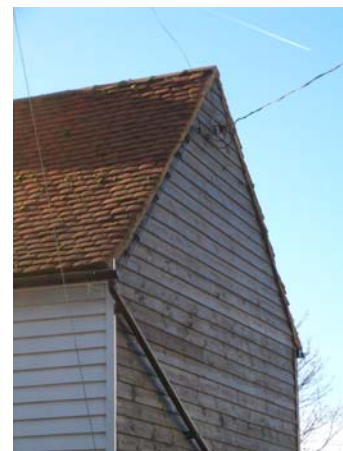
Fig. 13, Steep plain tile roof, with weatherboard painted white to front and black to sides and rear
