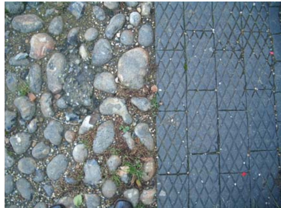
Fig. 21, Flint and blue stable block floor covering
