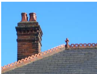
Fig. 14, Natural slate roof with ornate ridge and hip tiles
