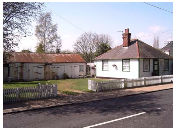
Fig. 19, Timber picket fence
