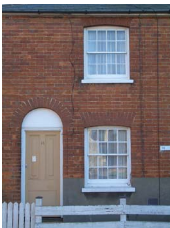
Fig. 11, Brick arches and timber joinery
