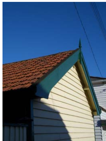
Fig. 15, Pan tile roofed outbuilding
