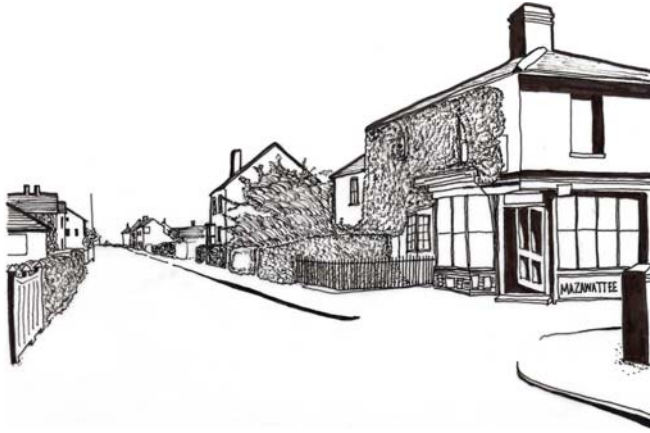
Fig. 33, South Street C.1910
