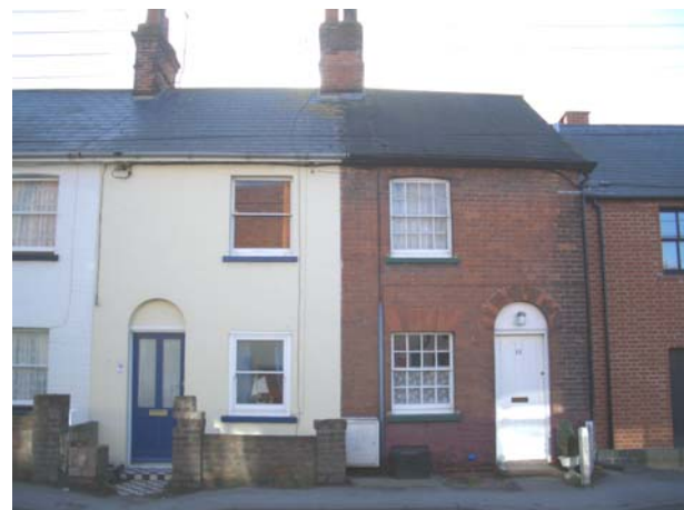
Fig. 20. Typical Victorian terrace
