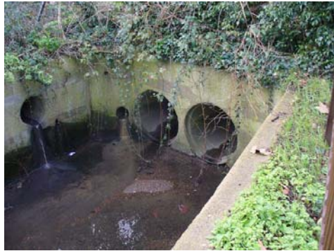
Plate 5-7 Culverts in a fluvial system. Note: the two smaller culverts are source from surface water drains
