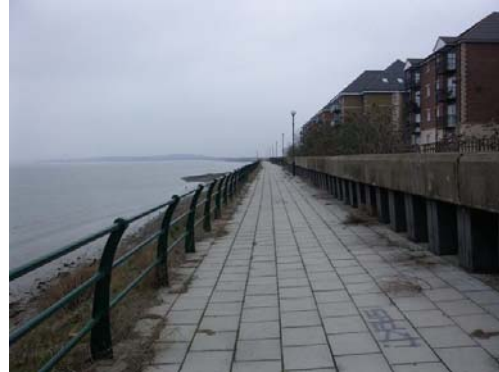
Plate 5-5 Example of sheet pile wall as a secondary flood defence
