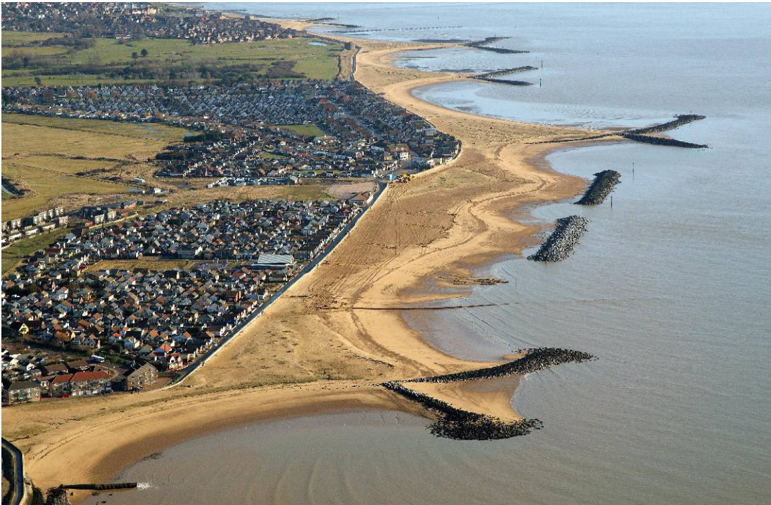
Figure 2-1 Coastal defences along the Tendring peninsula
