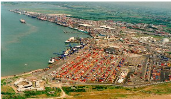
Figure 1-3 Felixstowe Port - northern boundary
