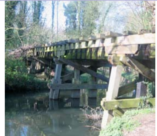
Fig 2F Timber Trestle Viaduct
