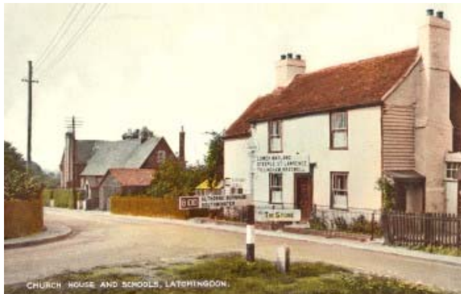
Church House and Schools, Latchingdon
